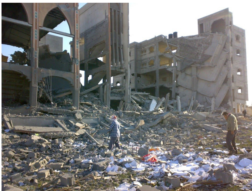
Figure 17-1. A building destroyed in Rafah during Operation Cast Lead.
