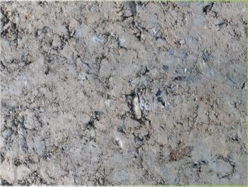
In these pictures we have the roller standing by ready to compact the DSA down to the proper compaction after the DSA has been laid down. The second you can see the DSA after compaction showing tell tale signs of proper compaction. When the DSA is at it's maximum compaction the larger stones that are in the mix can start to shatter. This can be noted by the slightly lighter grey color at the surface.
