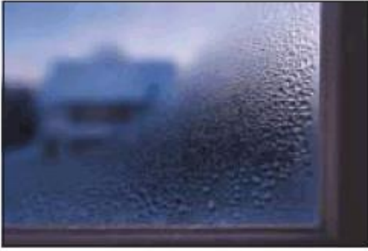
Condensation on the inside of a windowpane.
