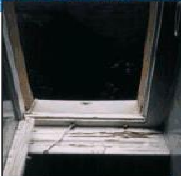
Leaky window — mold is beginning to rot the wooden frame and windowsill.
