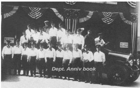
The first piece of motorized fire equipment was a 1921 Mack hose and chemical truck. It had no pump, but a fire extinguishing agent could be sprayed from its chemical tank through a hose reel. It carried hand tools, nozzles, and ladders as well as fire hose and was in service until 1936.
