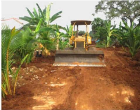
The ground behind the house is broken and must be filled with earth
