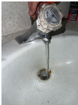
Deficient sink stopper, rust in sink
