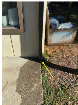
Downspout terminates at foundation
