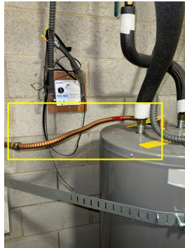
Flexible copper TPR discharge tube
