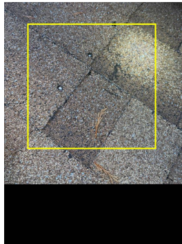
Damaged shingles
