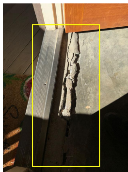
Large cracking
