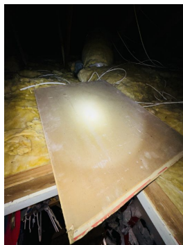
Uninsulated attic hatch
