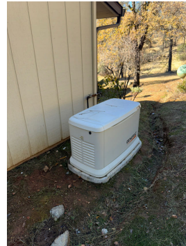
Auxiliary generator system not inspected
