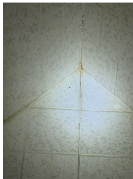
Cracked grout
