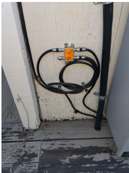
Deficient paint on siding
