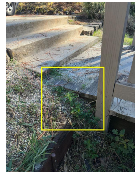
Deck structure to earth contact
