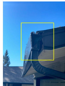
Damaged gutter
