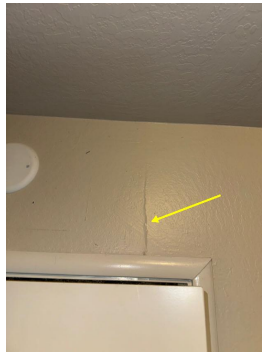
Sheetrock crack
