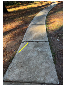
Walkway crack
