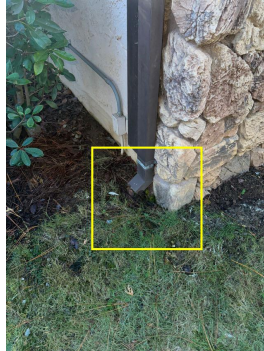
Downspout terminates at foundation
