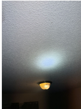
Room 8 popcorn ceiling texturing
