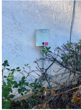
Septic system not inspected
