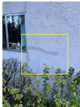
Patched stucco cracks, left side
