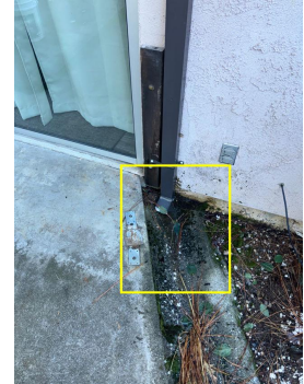
Downspout terminates at foundation
