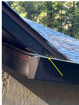
Barge rafter to roof contact, left side
