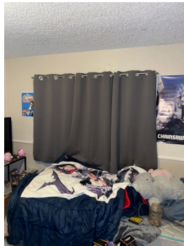
Room 9 blocked window
