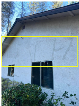
Patched stucco cracks , left side
