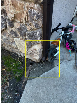
Downspout terminates at foundation
