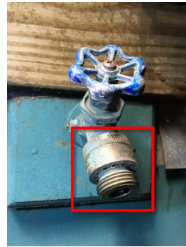
Example of an anti siphon vacuum breaker
