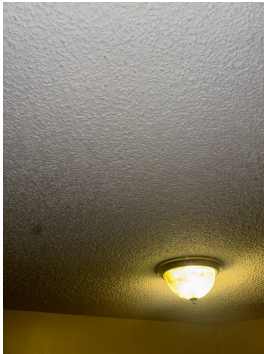
Room 9 popcorn ceiling texturing
