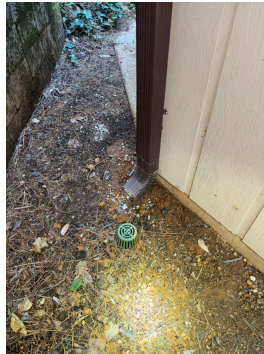
Downspout terminates at foundation with drainage system
