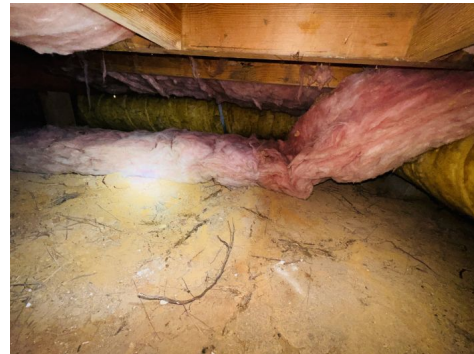
Disturbed insulation
