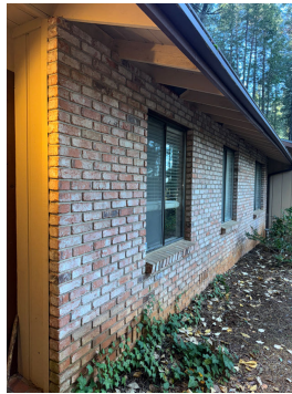
Masonry veneer without drain plane
