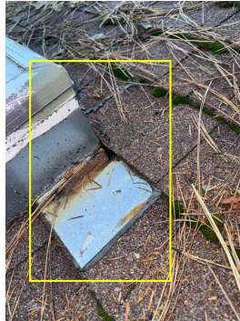
Mastic sealant around skylight flashing
