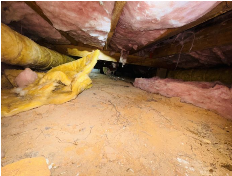
Disturbed insulation
