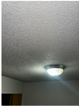
Room 2 popcorn ceiling texturing
