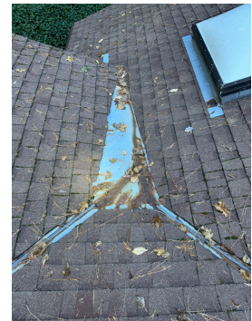
Rusted flashing
