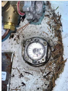
Gas tank at 10%
