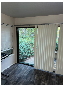
Sliding glass door difficult to operate
