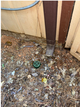
Downspout terminates at foundation with drainage system
