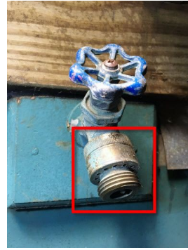
Example of an anti siphon vacuum breaker
