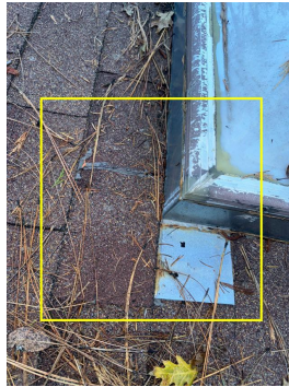
Mastic sealant around skylight flashing
