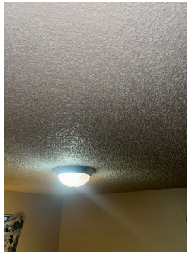
Room 3 popcorn ceiling texturing
