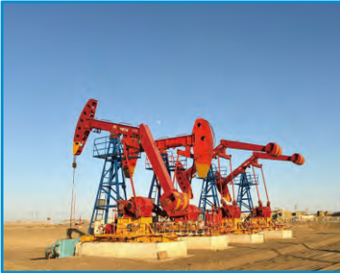
Oil production equipment
