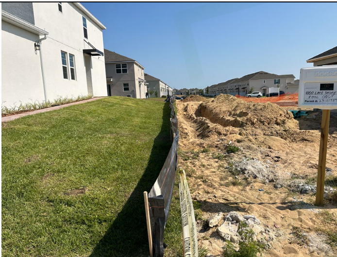
Site Conditions - Removed and hauled off a total of 65 truck loads of dirt - Can't run cabana sewer or start pool deck until the grading is resolved
