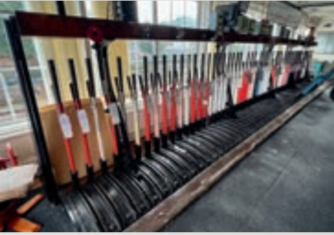
▲ In October Bridlington became one of the latest locations to lose its semaphore signalling in favour of colour lights, with a new control panel fitted inside the North Eastern Railway signalbox. However, the steam-era lever frame has been retained for posterity inside the Grade-II Listed building from 1893. Network Rail
