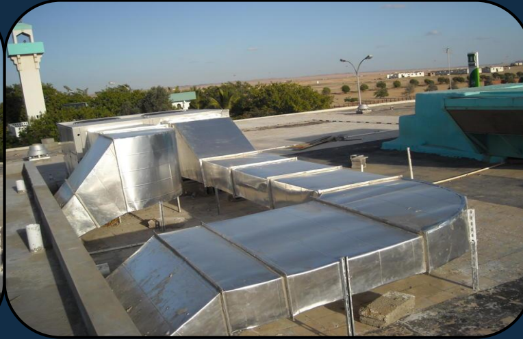
HVAC System: AC Ductwork [Project: Taif Airport]
