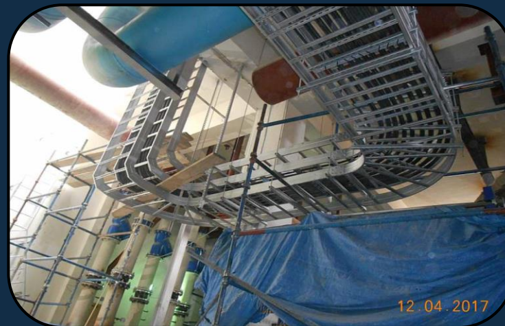
Cable Tray Arrangement
