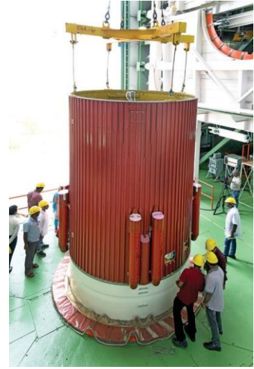
Placement of interstage over PSLV-C55 first stage during vehicle integration
