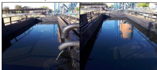
API Separator with NX Chemical Treatment
