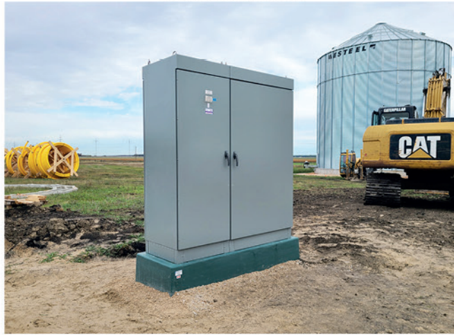
1200A Switchboard, Manitoba, June 2023
