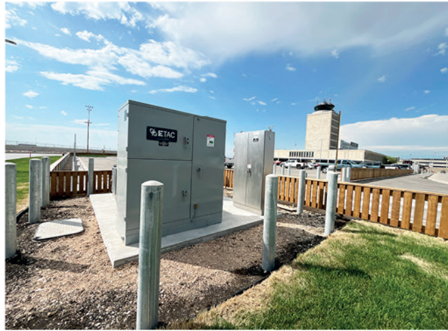
750kVA Visible Break Transformer & 800A Panel, Winnipeg, June 2025
