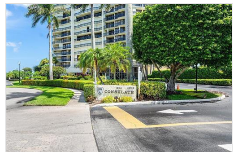
THE CONSULATE DRIVEWAY
