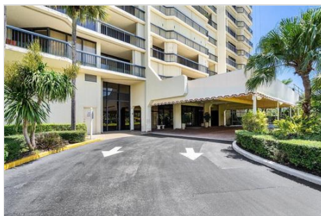
THE CONSULATE DRIVEWAY
