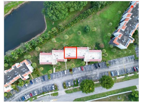
Building Above Unitt Location
