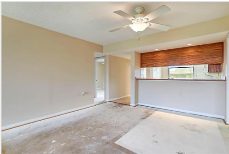
Entrance to the Second Bedroom
