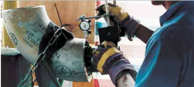
An elbow mandrel head being mounted in a fitting and being aligned with a dial indicator for maximum precision.
