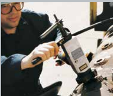
The rugged, ratchet feed, BOILERMASTER seen rapidly facing torch-cut header stubs.
