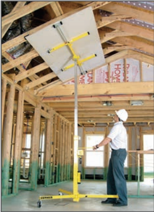
The platform tilts up to 45° for cathedral-type ceilings
