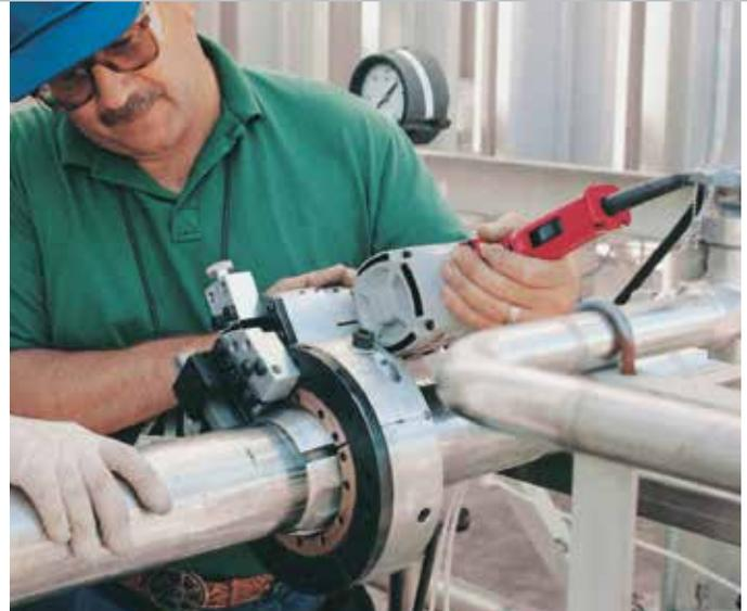
A piping system contractor performing outage maintenance on thin-wall stainless piping system uses an electrically powered SB clamshell fitted with full support pads. The piping system was part of an auxiliary high purity nitrogen supply line at a semiconductor manufacturing facility. A prefabricated pipe assembly was then orbitally welded in place without any additional end-prep being required.
