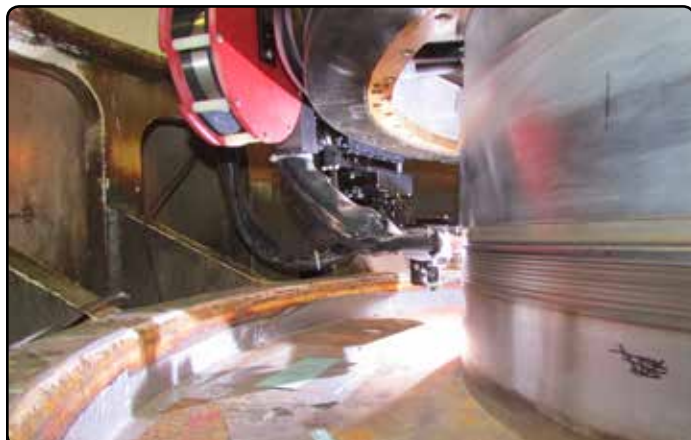
Turbine shaft cutout, AdaptARC reweld, and re-machine repair for a power plant.
