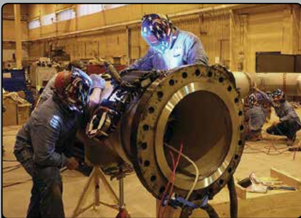
AdaptARC equipment doing WPS development in a Geothermal plant.
