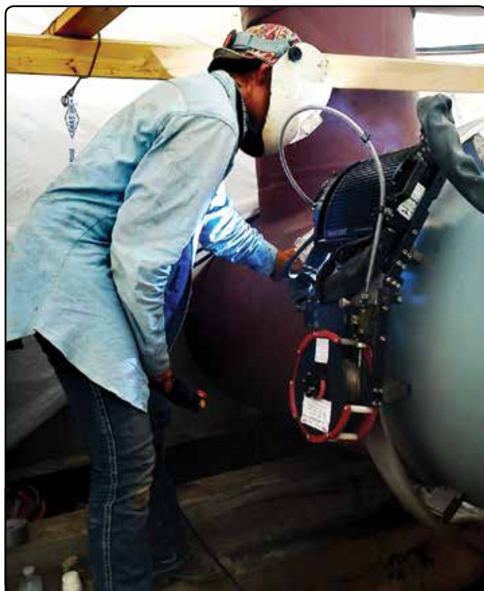
High performance AdaptARC welder in operation at Marcellus Oil & Gas Project.
