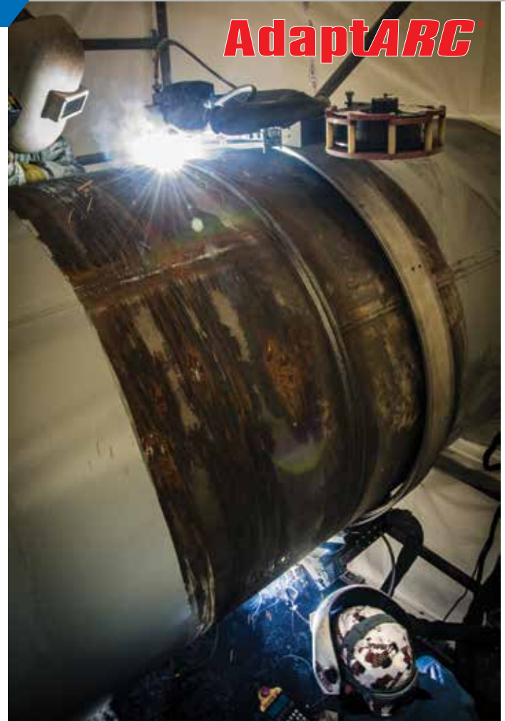
Two Tri Tool DualARC orbital weld heads operating simultaneously on a single mounting track for maximum weld deposition on an onshore LNG project.
