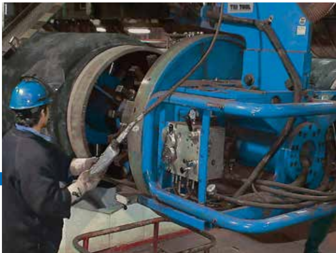
Tri Tool's powerful PIPEMASTER PFM 3248 is being positioned into the end of a concrete lined pipeline section prior to performing weld end preparation.
