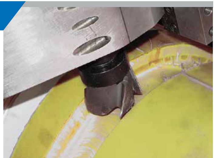
This section of offshore coated pipe is having the outer two layers of coating removed with an in-line, OD mounting split frame lathe.
