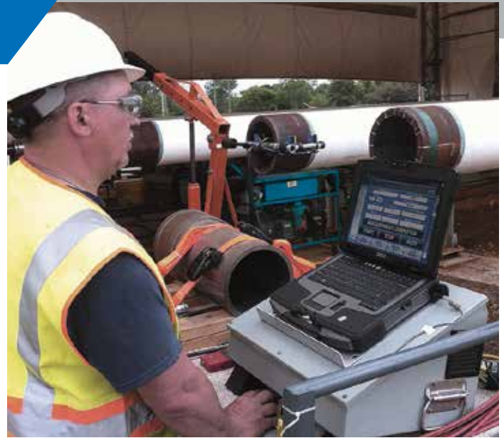
Tri Tool's Laser Dimensioning System records precise measurements of each pipe end so that ends can be accurately matched for improved welding results.
