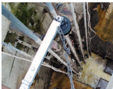
RETENTION TANK WITH SMALL CLUTTERED WET WELL AT 15m
