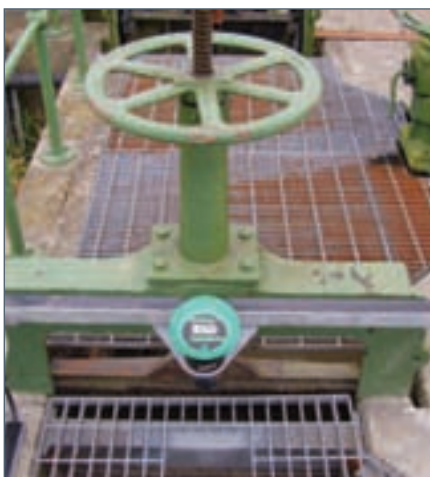
IMP CONTROLLING SCREEN HEIGHT
