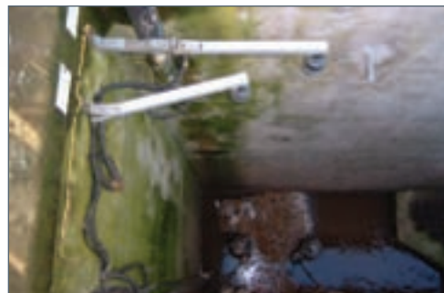
HINGED BRACKET OVER A WET WELL
