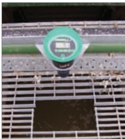
IMP CONTROLLING GATE HEIGHT
