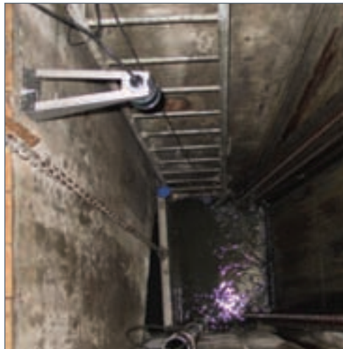
WETWELL 6m WITH LADDER AND FLOAT
