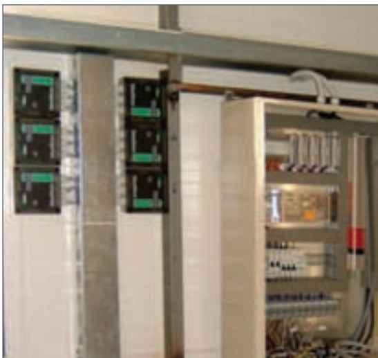
MINERAL OIL TANK LEVEL
