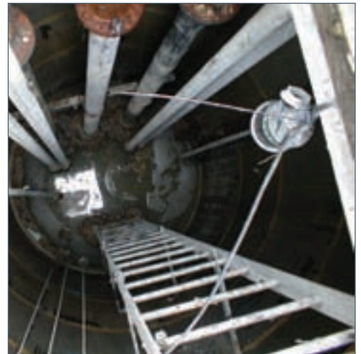
WETWELL 4.5m WITH LADDER AND FAT RING
