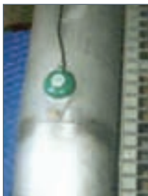
2010 SENSORS FITTED TO ANIMAL FEED CHUTES
