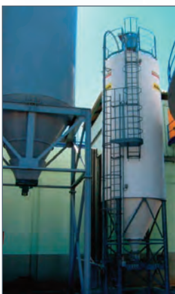
UltraTWIN with dB10 and dB15 on 7m (23ft) and 10m (33ft) silos containing powder
