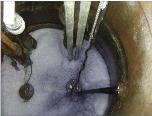
3.5m (11ft) FOAMY WET WELL PUMP CONTROL
