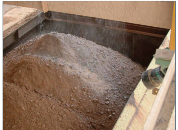
RAIL TRUCK LEVEL FOR WATER SPRAY CONTROL
