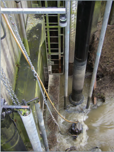
7m (23ft) PUMP CONTROL
