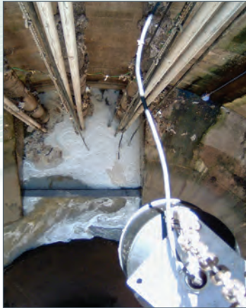
27m (89ft) STORM TANK 3 PUMPS DOWN CENTRAL WELL
