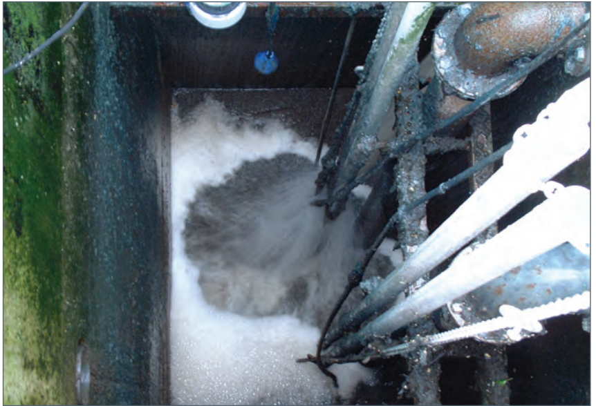
4m (13ft) WET WELL PUMP CONTROL AND HIGH FILL RATE
