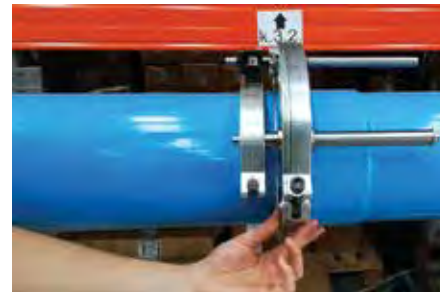
Step 6: Release UnipipeEZ Install Tool from pipe.
