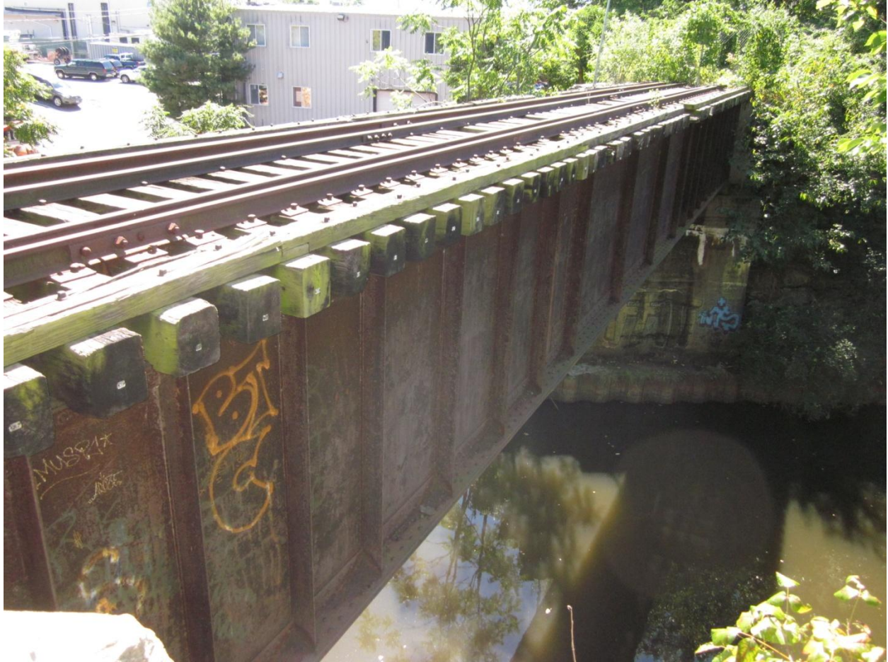
Figure 13: Charles River Bridge Crossing
