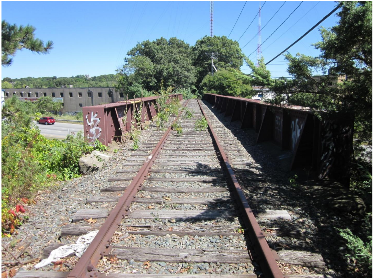
Figure 15: Route 128/I-95 Crossing
