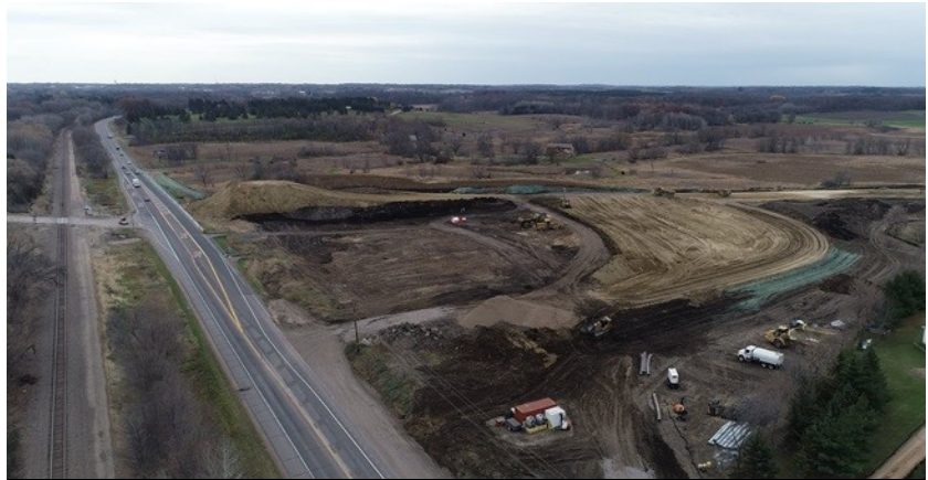
View of the construction area south of Highway 12, where the roadways are being realigned and work on the new bridge has begun.
