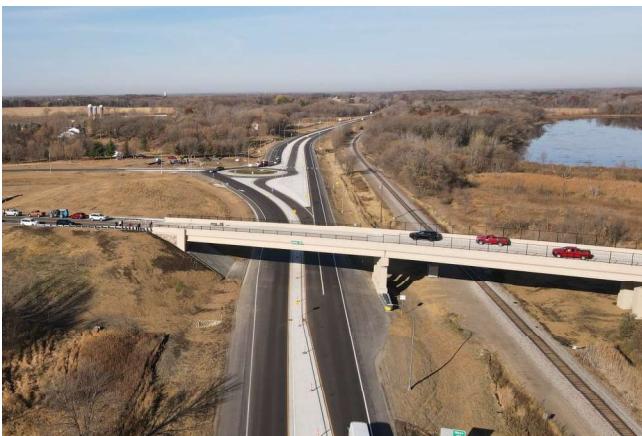
Aerial views of the redesigned intersection, round-a-bout, and County Road 92 overpass at Highway 12
