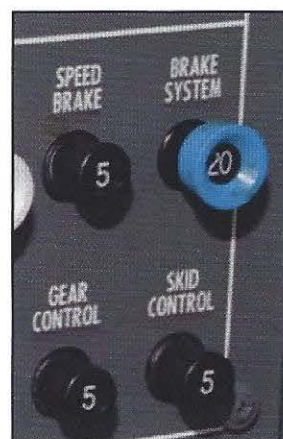
Figure 5-29: Anti-Skid Control Circuit Breakers
