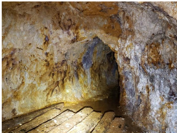
Left Photo: Inside the adit at the 40-meter mark. Boards cover flooded winze. Right Photo: Left crosscut, sericitized zone.
