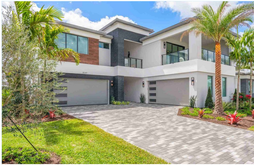
Luxury New Construction — Palm Beach County
