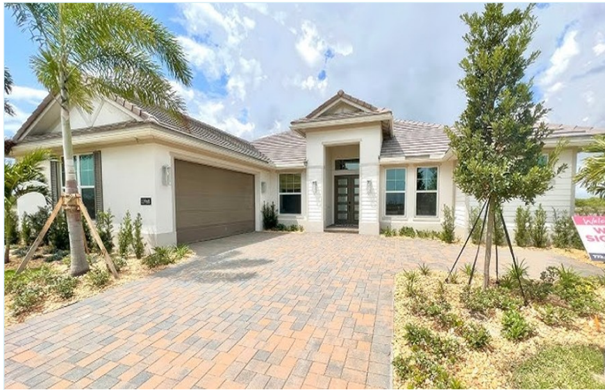
New Construction — Belterra, Port St. Lucie
