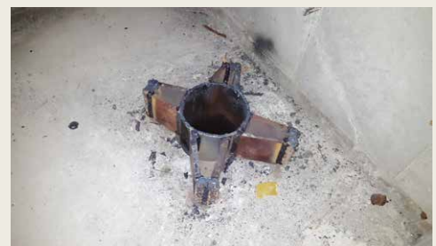
Pressed pile installation-exposure on the foundation
