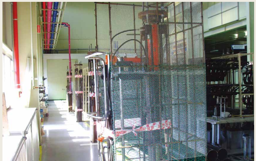
The first construction | foundation reinforcement reconstruction
