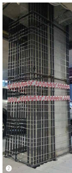
Details of Steel plate Column reinforcement with epoxy bonded
