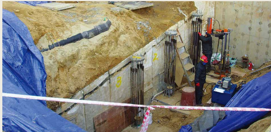
Under construction | top foundation reinforcement, settlement, joint hole, pile, basement reinforcement
