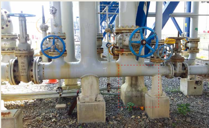
Column foundation reinforcement within dotted line
