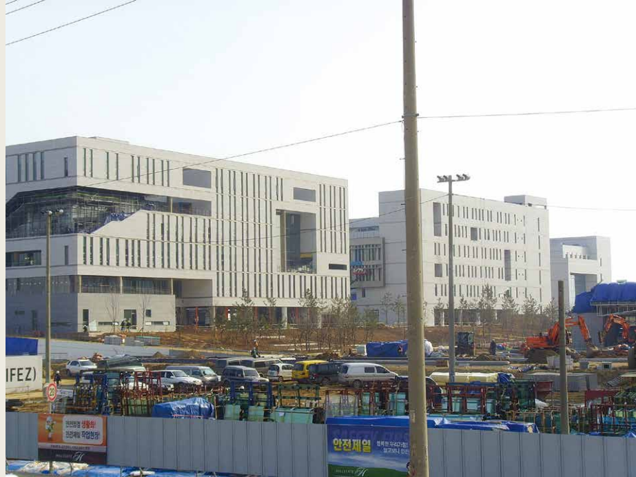
The front view of building under construction
