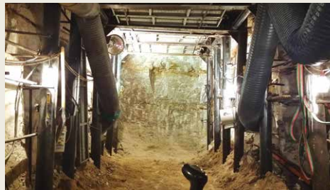
Underground joint hole 90m underground tunnel connection work
