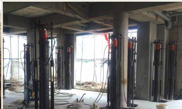
Under construction of pressing piles
