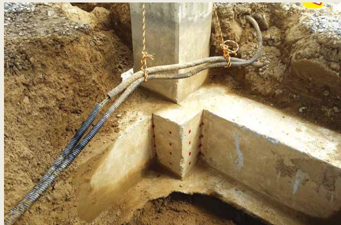
Foundation reinforcement after the increase of the cross section by reinforcing shearing bar
