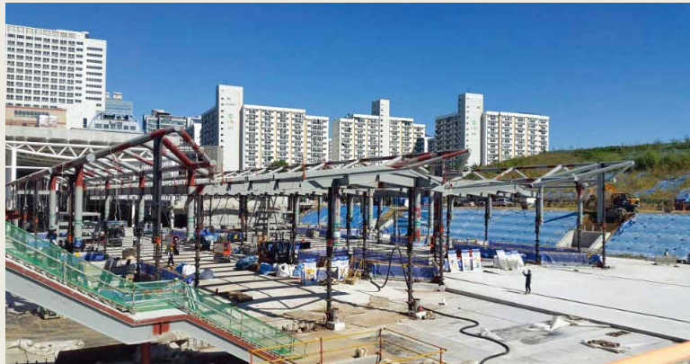
After column cutting 3m and raising
