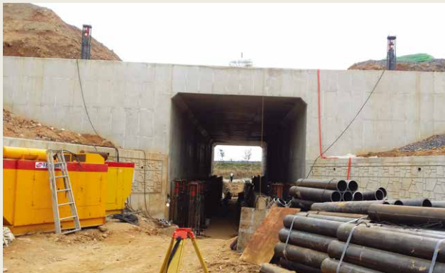
Under construction of settlement box
