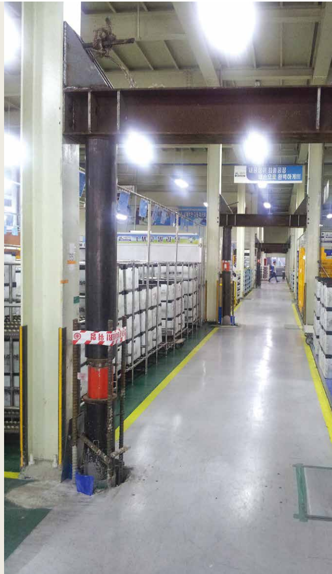
The second construction | foundation reinforcement during operation of automobile parts company
