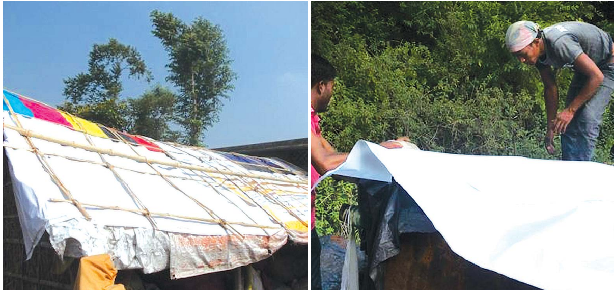
Figure 35. Utilization of the Flex Banners to Cover the Tin-Roofed Shanties [24]
