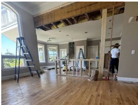
4 Replacement structure installed and opening formed.
