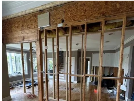
2 Load path and field conditions verified; utilities coordinated.
