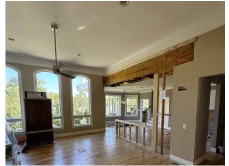
3 Temporary support and structural installation prepared.
