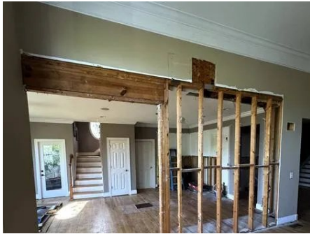
1 Existing finishes removed and structural framing exposed.
