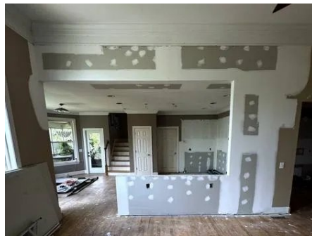
5 Framing enclosed and the space prepared for finish work.
