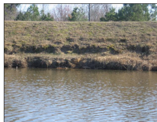
Dam embankment eroded by storm water, June 2008.
