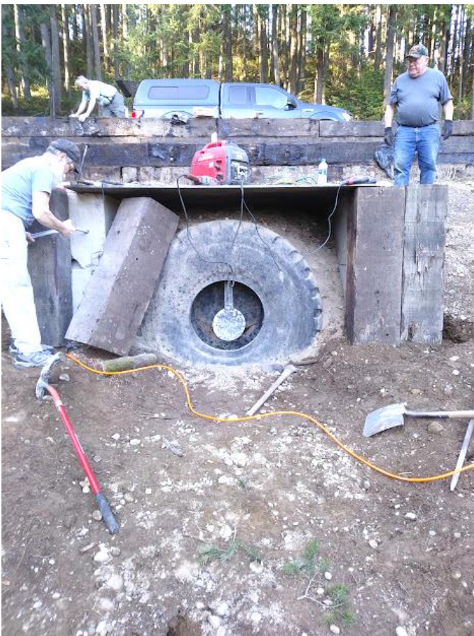
Mark Voigt, Ed Cole and Darrell Behounek hard at work Photos courtesy of Mark Kosin
