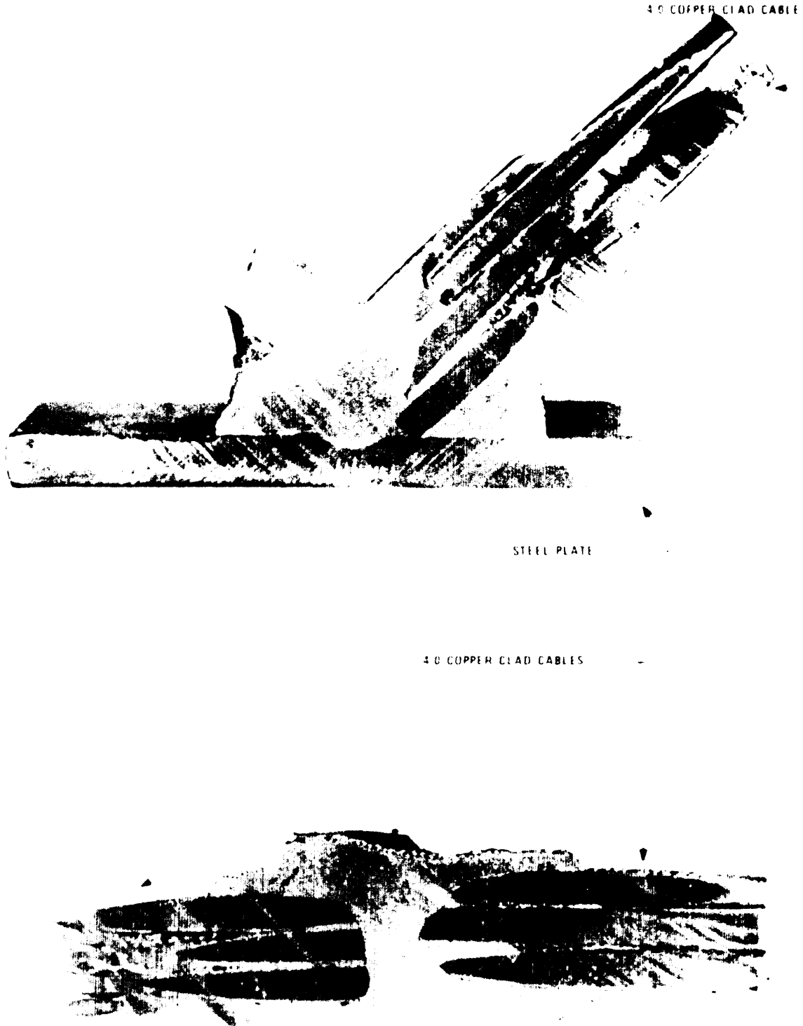
Figure 7-5. Typical Exothermic Connections
