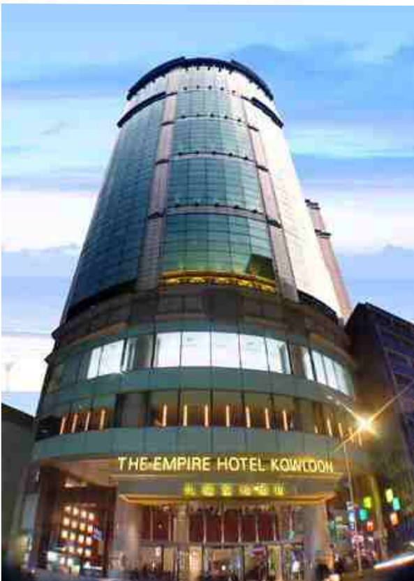
Empire Hotel Kowloon • Tsim Sha Tsui - Hong Kong, China
