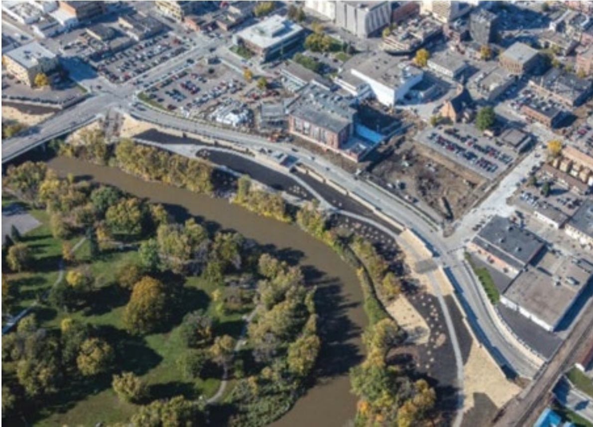
Photo: Fargo-Moorhead Flood Risk Management project; estimated federal cost savings from public-private partnership: $100M
