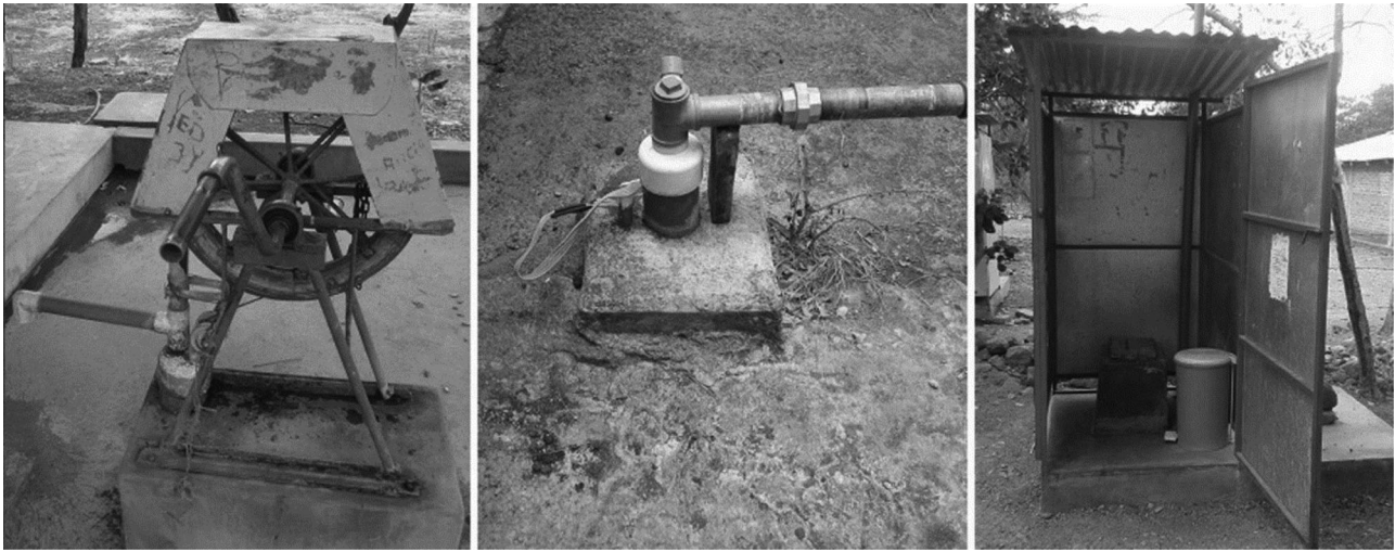
Figure 1. The three primary WatSan technologies in Darío. Rope and electric pumped wells (left and middle, respectively) and ventilated improved pit latrine (right).
