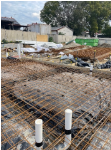
Figure 5 Typical slab for better ground conditions (note the reduction in reinforcement)
