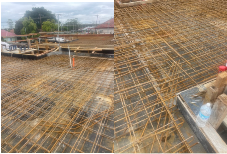
Figure 9 First floor construction photos of the first-floor slab prior to placing concrete
