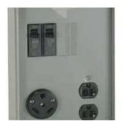
When you get to the campground, you will find an electrical box such as this. Shut off all breakers, plug in the camper, then turn breakers on. Use the 3 prong 30amp plugin.
