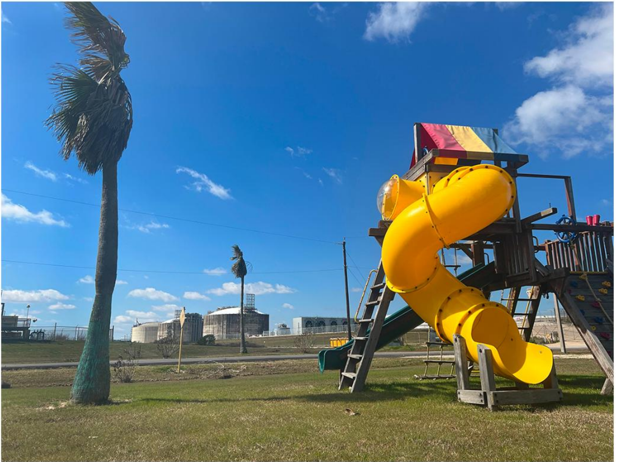
A playground is pictured near storage tanks for Freeport LNG's export terminal in 2023. | Shelby Webb/POLITICO's E&E News
