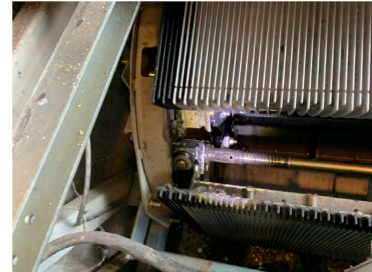
Step chains appear to be well lubricated, and no damaged rollers or step axles were found during the visual inspection
