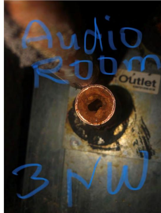
*Chilled water scaling build-up within fan coil unit*
