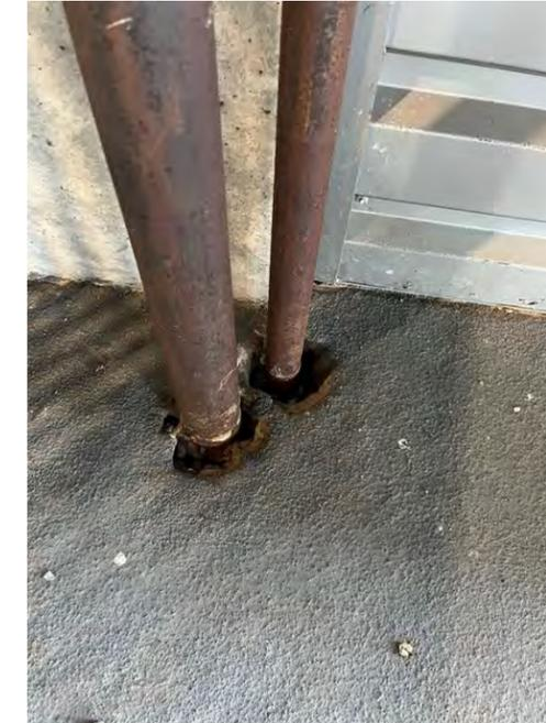
Corrosion on piping exterior and missing slab penetration sleeve/collar
