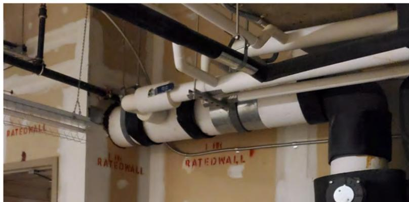
Fire proof caulking not observed at plumbing penetrations through rated walls
