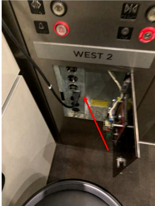
Fans are plugged into the car operating panel behind inspection doors
