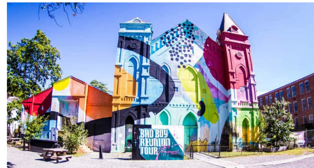
Washington DC adaptive reuse of existing church. Example of using existing buildings and giving them a new life through art.
