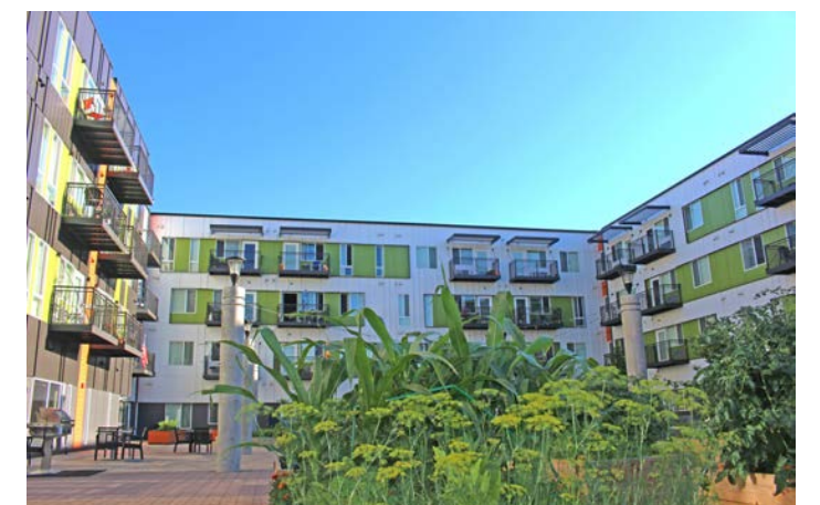
Belmar Metro West Housing- interior courtyard
