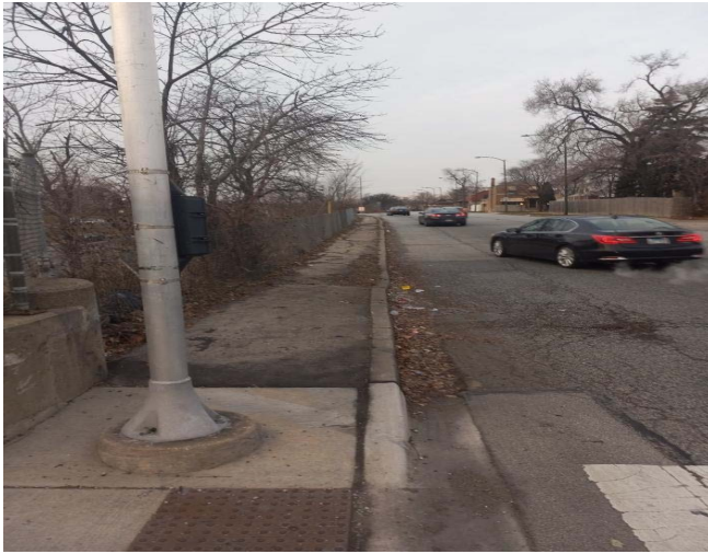
99 TH / HALSTED S/B ENTRANCE RAMP BEFORE
