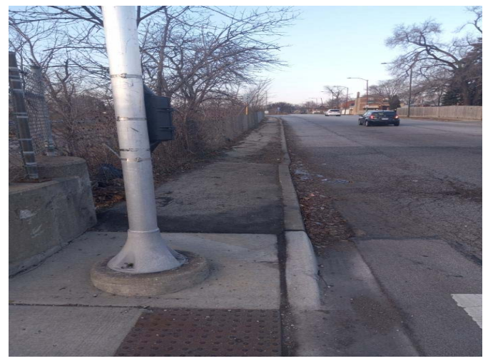
99 TH / HALSTED S/B ENTRANCE RAMP AFTER
