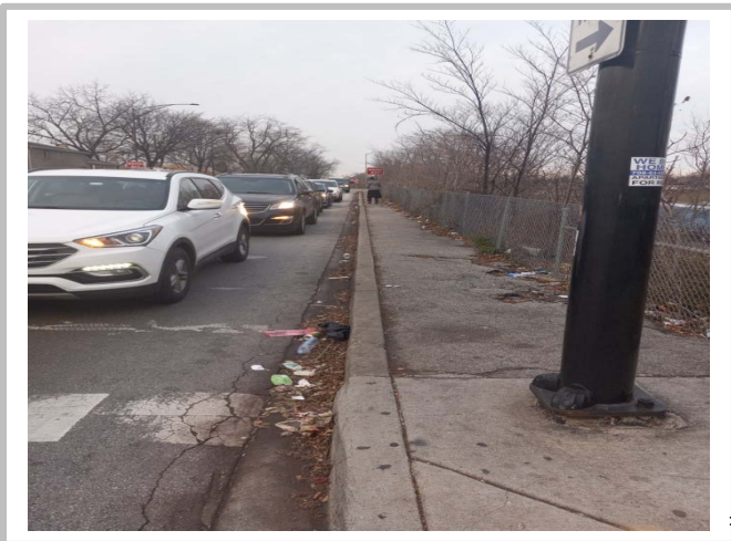
99 TH / HALSTED N/B EXIT RAMP
