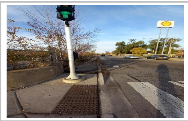
99 TH / HALSTED SB ENTRANCE RAMP BEFORE
