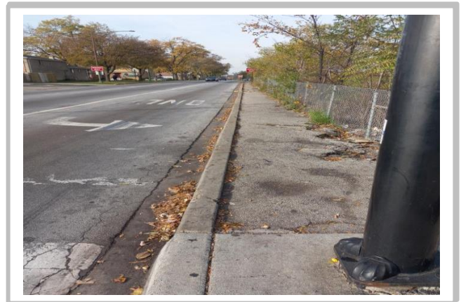
99 TH / HALSTED NB EXIT RAMP AFTER
