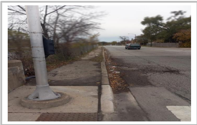
99 TH / HALSTED SB ENTRANCE RAMP BEFORE
