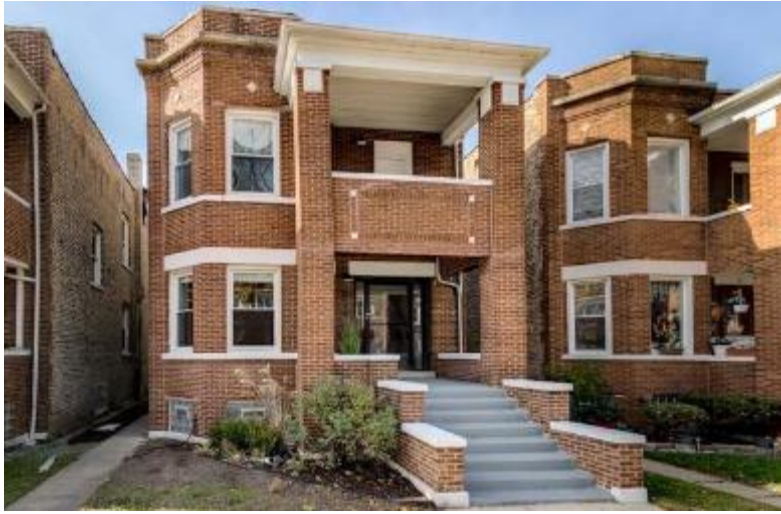
LOW DENSITY - TWO & THREE FLAT REHAB
